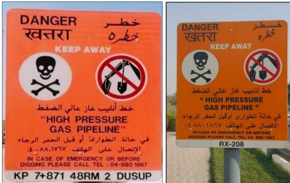
Figure 2 DUSUP Pipeline Warning Sign with KP Numbers and DUSUP Pipeline or Road Crossing Number (RX or DX) – Emergency Number
