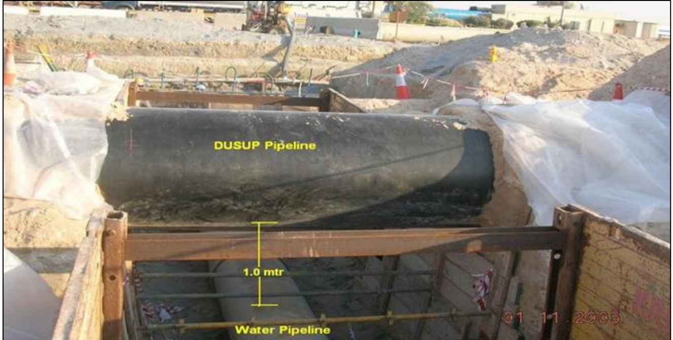
WATER PIPELINE CROSSING UNDERNEATH DUSUP PIPELINE – OPEN CUT
