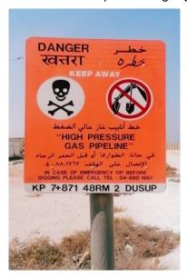
The spacing of signs may be reduced to suit site conditions such as in JAFZA or to indicate a change of pipeline direction.
