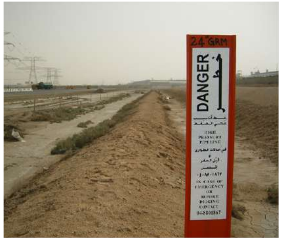
DUSUP PIPELINE MARKERS
