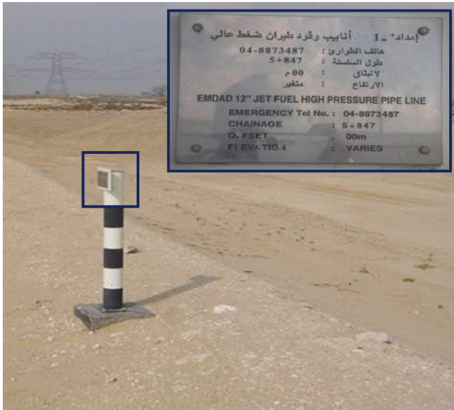
EMDAD berm and Warning Sign
