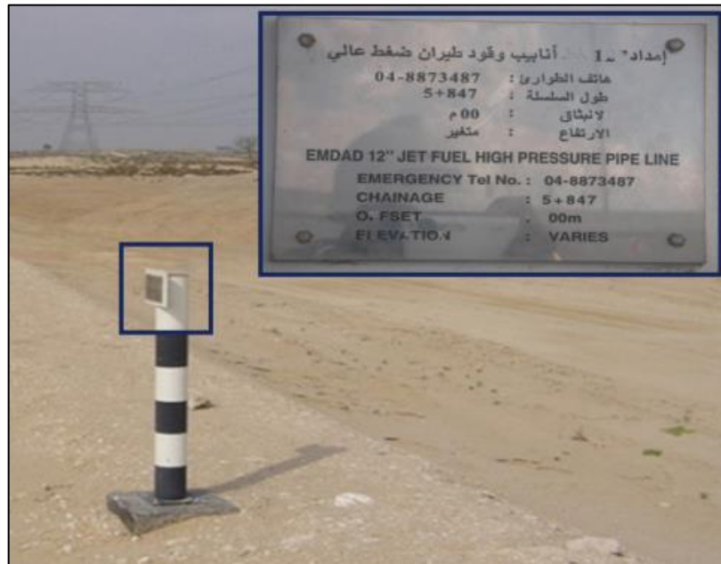
Figure 3 EMDAD Warning Sign
